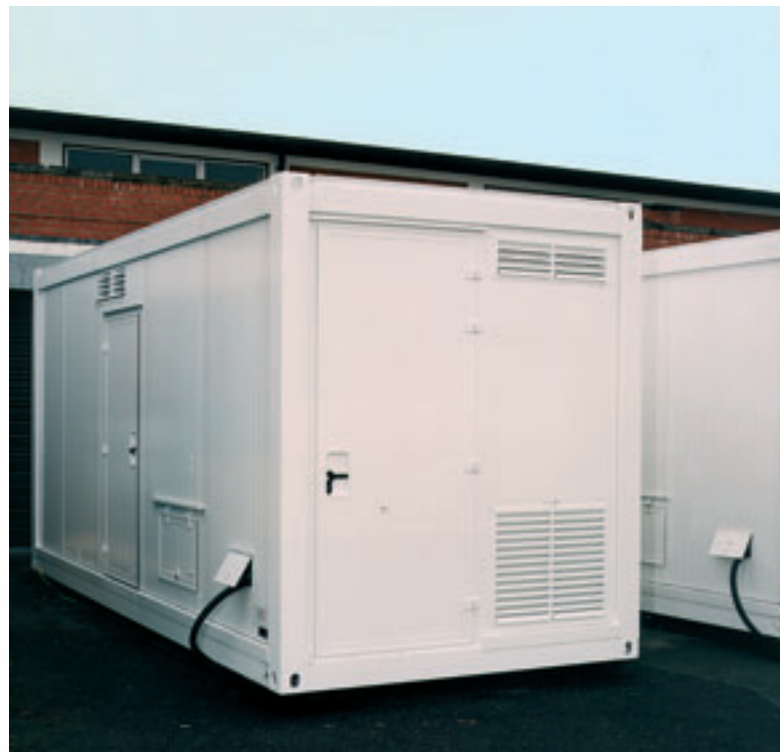
Compact and mobile – each of these containers houses a complete 20 kW TV transmitter.
